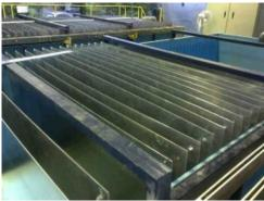
WWTP Electrocoagulation system at Automotive Manufacturing Plant at East Jakarta with Capacity 200 M³ per day:
