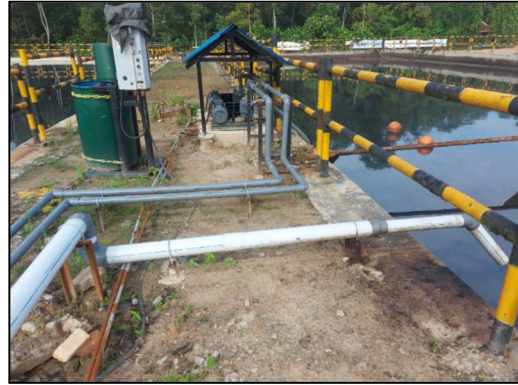
Sistem Perpipaan Pompa Intake
